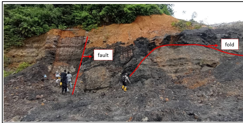
Figure 4. Folding and faulting in coal seams in the Merangin area, Jambi, highlighted in red in the image (Photograph by Rakhmatul Arafat, Tabir Ulu, Jambi, Indonesia, 2025).
